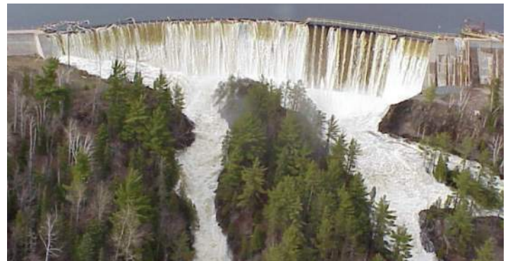
Hoist Dam — Dead River Storage Basin
