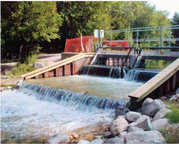
Glen Lake Dam in Leelanau County
