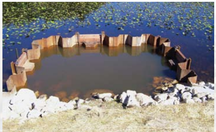
Lake Level Control structure for upper Crooked Lake in Barry County
